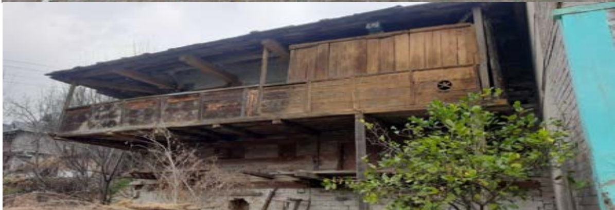
Traditional wooden houses with kath kuni techniques and slate stone roof
